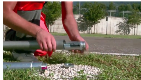
3. Insert expander into upper pole
