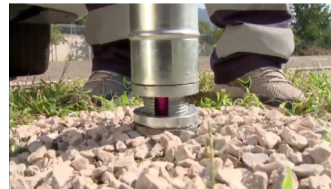
4. Spin SmartFlex into ground sleeve & upper pole
