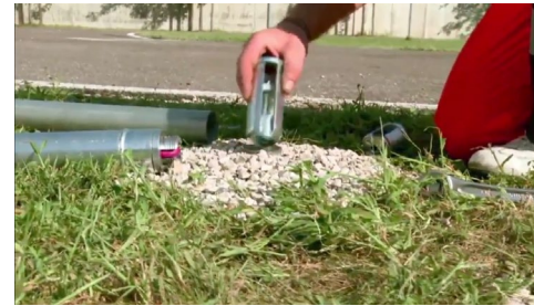
2. Insert expander into ground sleeve
